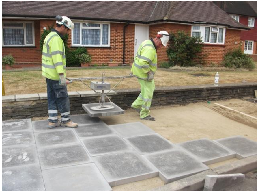
Crews carrying out paving works are working collaboratively with Virgin Media
