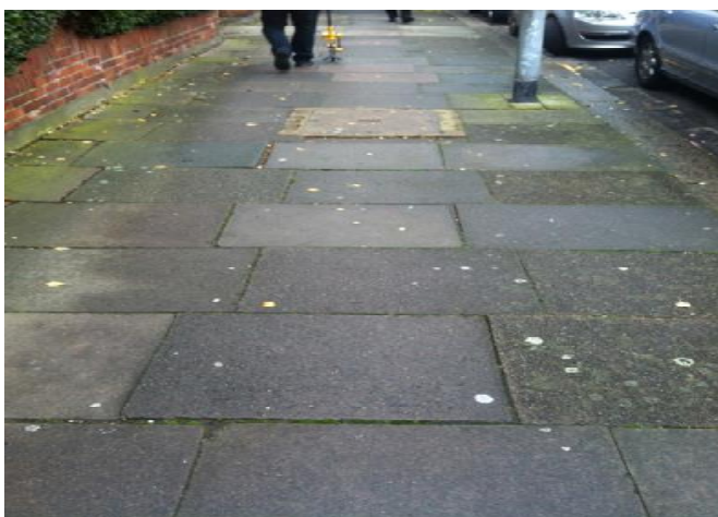
BEFORE: Stamford Brook pavement
