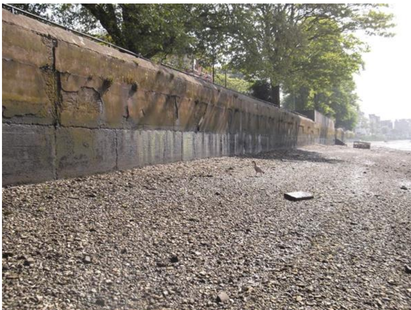
The retaining wall at Strand on the Green will be repaired over the next five months.
