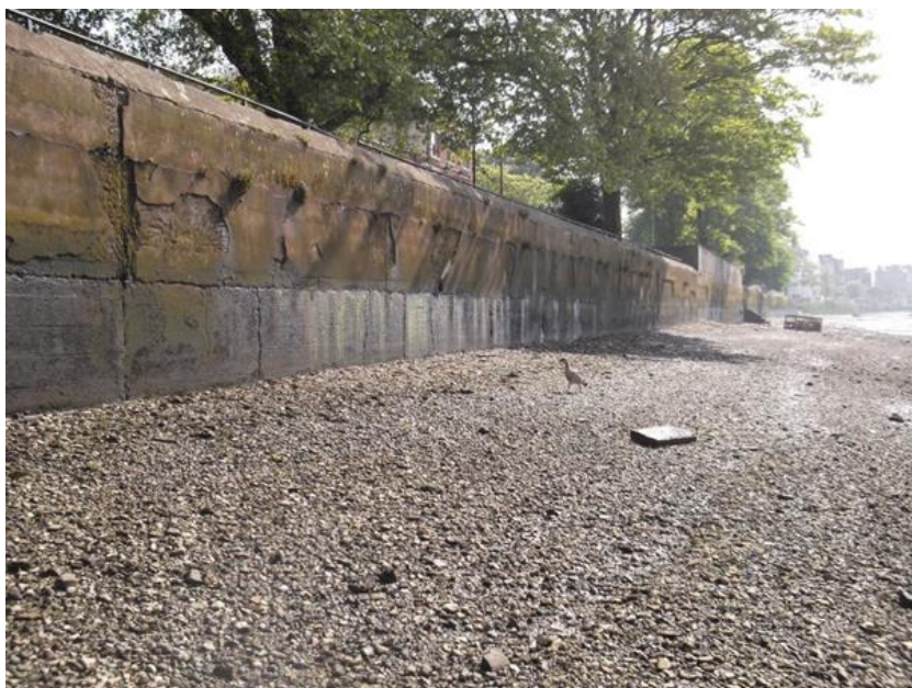
The retaining wall at Strand on the Green will be repaired over the next five months.
