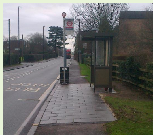
Completed footway works at a bus stop in Staines Road
