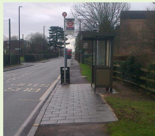
Completed footway works at a bus stop in Staines Road
