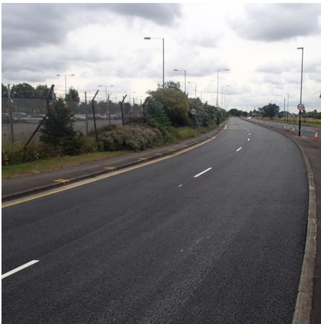
Hounslow Highways completed a major scheme on Stanwell Road East.
